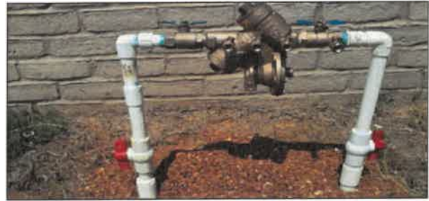
Example Installation of Irrigation Backflow Preventer
